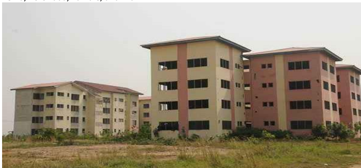
Figure 1. Borteyman affordable housing Project Abandoned in 2009
