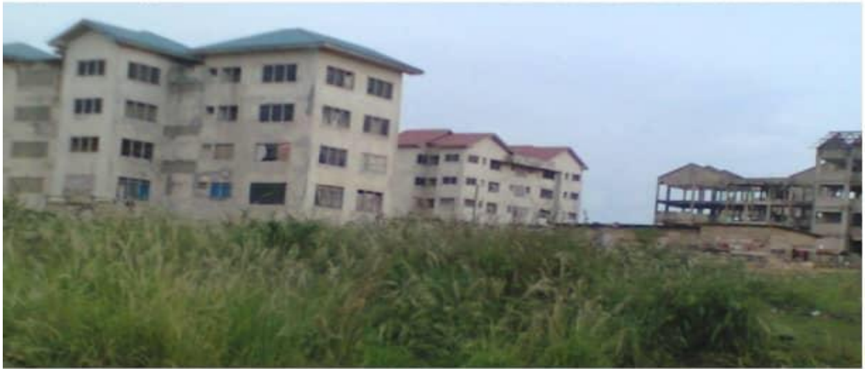
Figure 3. Asokore-Mampong Affordable Housing Project Abandoned in 2009
