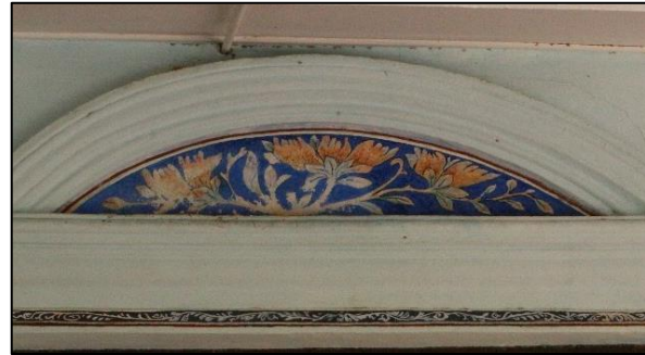
Figure 1.22: Decoration using chrysanthemum motif at the semi-circular arch panel Source: Field work
