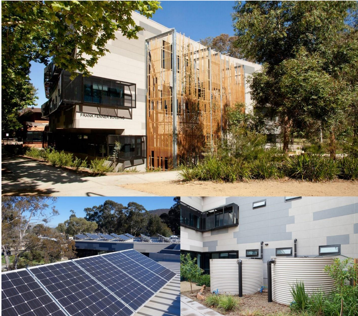
Figure 1: Frank Fenner Building, Fenner School of Environment and Society, ANU, showing views of solar panels on roof and the water recycling system (Australian National University, n.d.).
