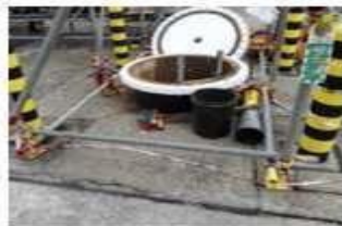
Confined space activity to do inspection work
