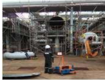
Manual handling to move material/equipment at site
