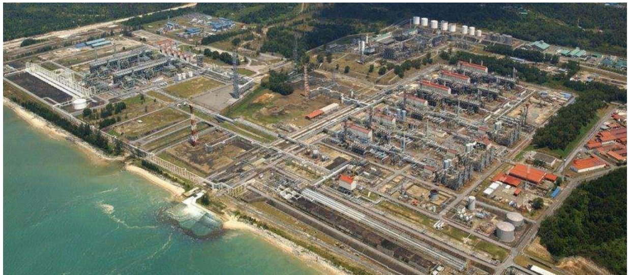
Figure 2 On-shore Plant Facility at Bintulu Sarawak Source: PETRONAS LNG Complex
