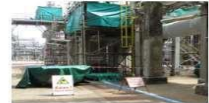
Hot work activity at height
