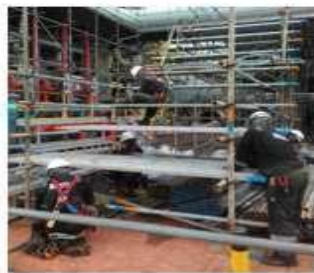
Erection of scaffolding as temporary platform
