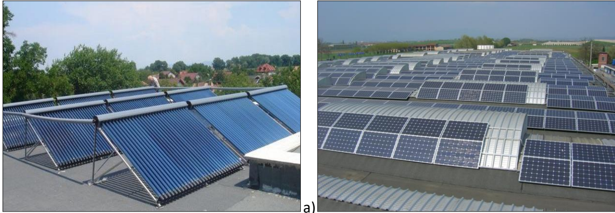
Figure 7. Installation of solar and photovoltaic panels for domestic hot water preparation
