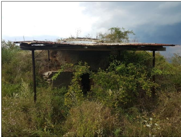
Figure 8. Lime kiln in ruins
