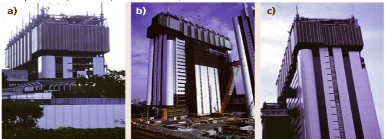
Figure 5 Obayashi Automated Building Construction System (ABCS) (a) early construction phase; (b) intermediate construction phase; (c) final construction phase adopted from (Saidi et al., 2016)
