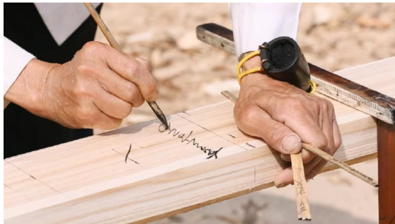
Figure 1. Zhang Mo Shi writes Mo Shi Wen to mark the position of the component in the entire building
