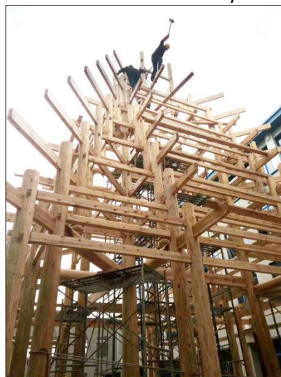
Figure 15. The wooden constructive structure of the Dong building
