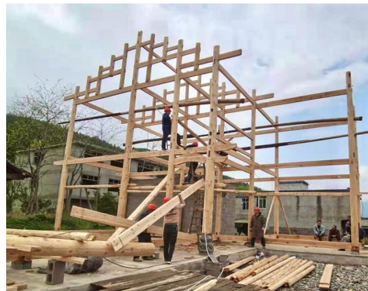
Figure 17. The Wooden Constructive Structure of the Dong Building
