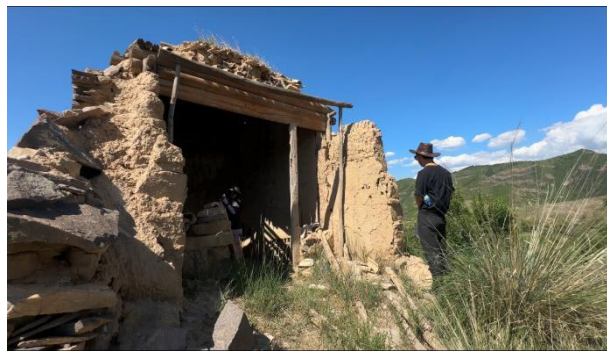
Figure 4. A broken mural (Source: Taken by the author in 16/6/2024)
