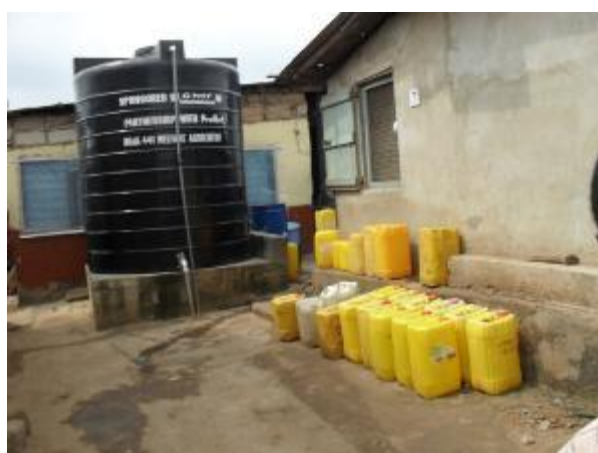
Fig. 2: Large water storage facility obtained through microfinance
