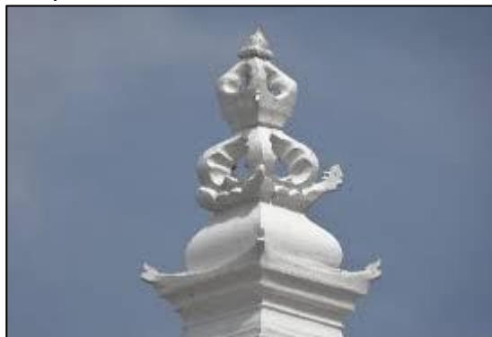
Figure 1.6: Roof Crown of Masjid Kampung Hulu
