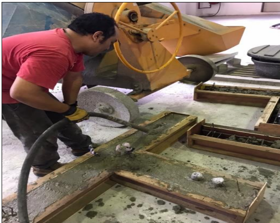
(c) Vibrating Concrete Process
