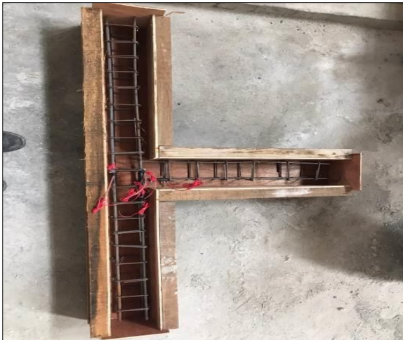
(a) Installing Reinforcement Bars in The Formwork
