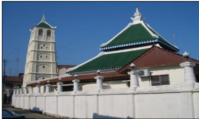
Figure 1.6: Masjid Kampung Keling with three tiers pyramidal roof
