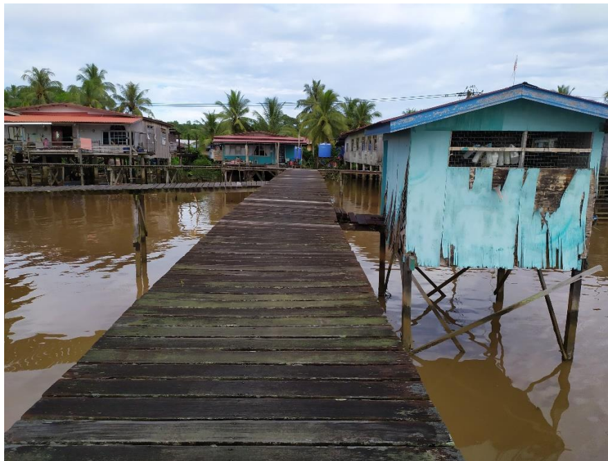
Figure 4 Footpath of the water village
